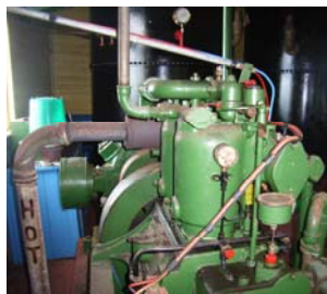
Gardner engine - drives the foghorn compressor
