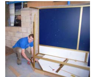
Showcases being installed
