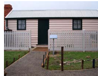
Pathways under construction
