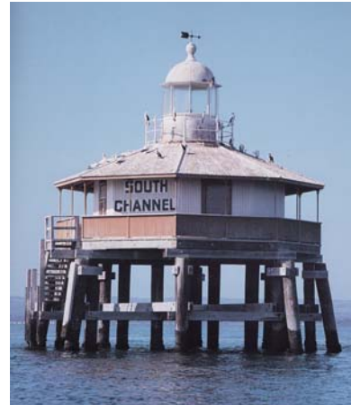
South Channel Pile Light rebuilt 1998
